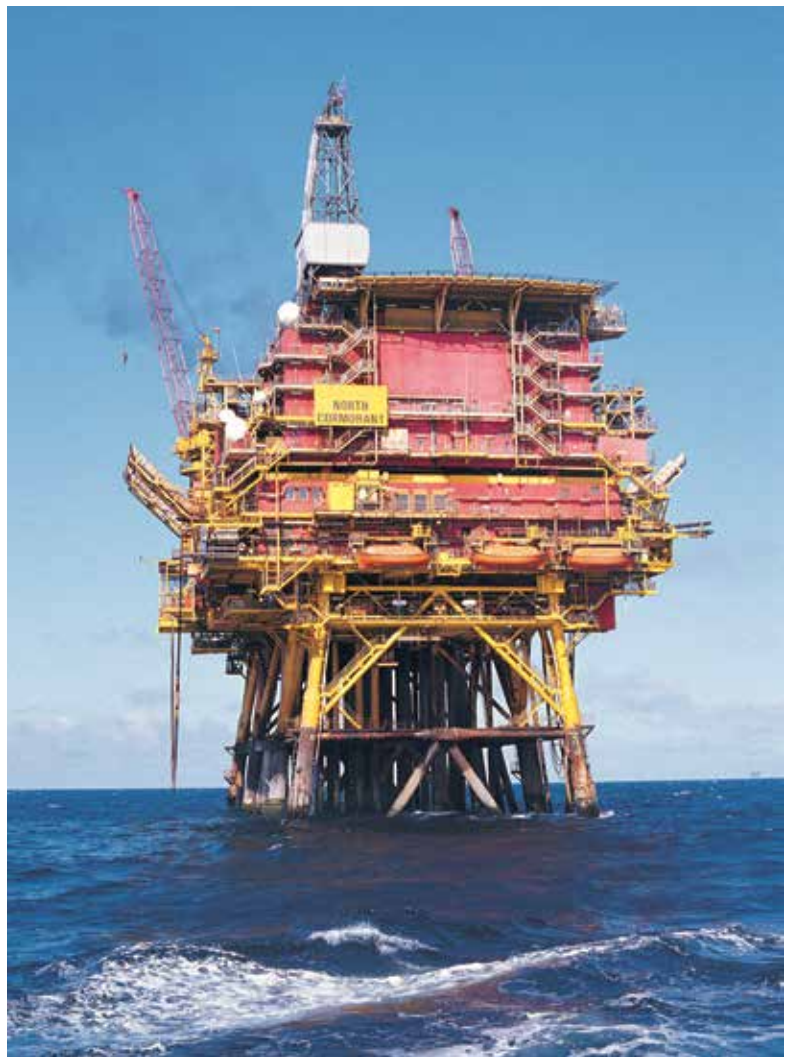
Figure 1: North Cormorant offshore platform, constructed in 1980, is in the East Shetland Basin of the northern North Sea. This visual indicator of a high-carbon lifestyle is in a remote location, approximately 110 miles north-east of Lerwick in the Shetland in water 161 metres deep.
