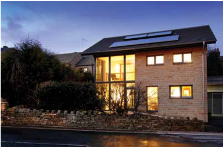
Figure 2: This three-bed detached house in Denby Dale, West Yorkshire is the first UK Passivhaus to be built with cavity wall construction. Its design relies on a simple tea cosy effect: with maximum use of super insulation and stringent levels of air-tightness. By combining this with optimum levels of ‘passive solar gain’ (heat from the sun) and Mechanical Ventilation with Heat Recovery systems, Passivhaus design can create healthy and comfortable buildings that require minimal heating. Photo: www.denbydalepassivhaus.co.uk
